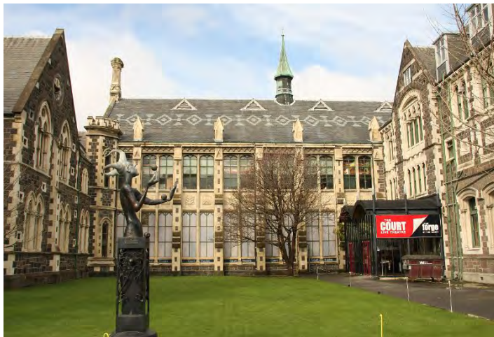
Figure 11 Arts Centre with original Court Theatre entrance
