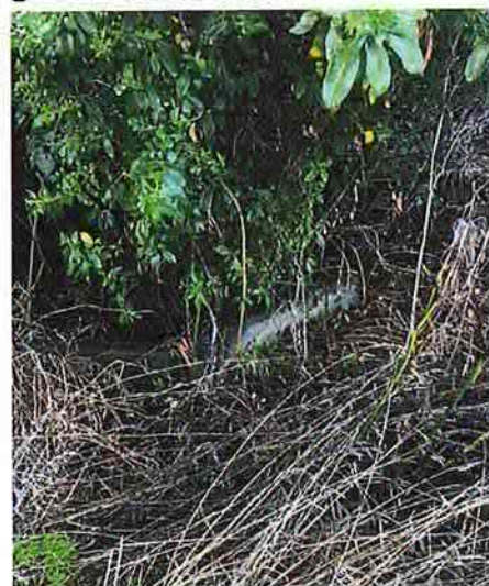
Over grown main storm water sump
