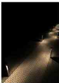
The Arch Bollard Ibeam (above left) has a low glare light fitting with precise light placement. 2700K but acceptable.
