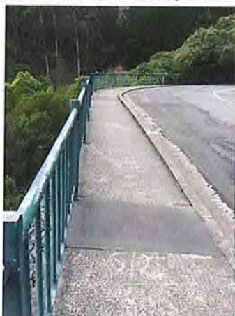
Kerb elevated above footpath
