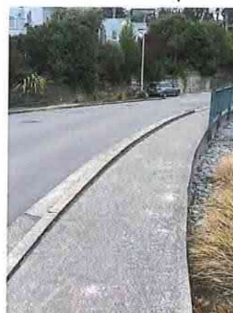
Kerb elevated above footpath
