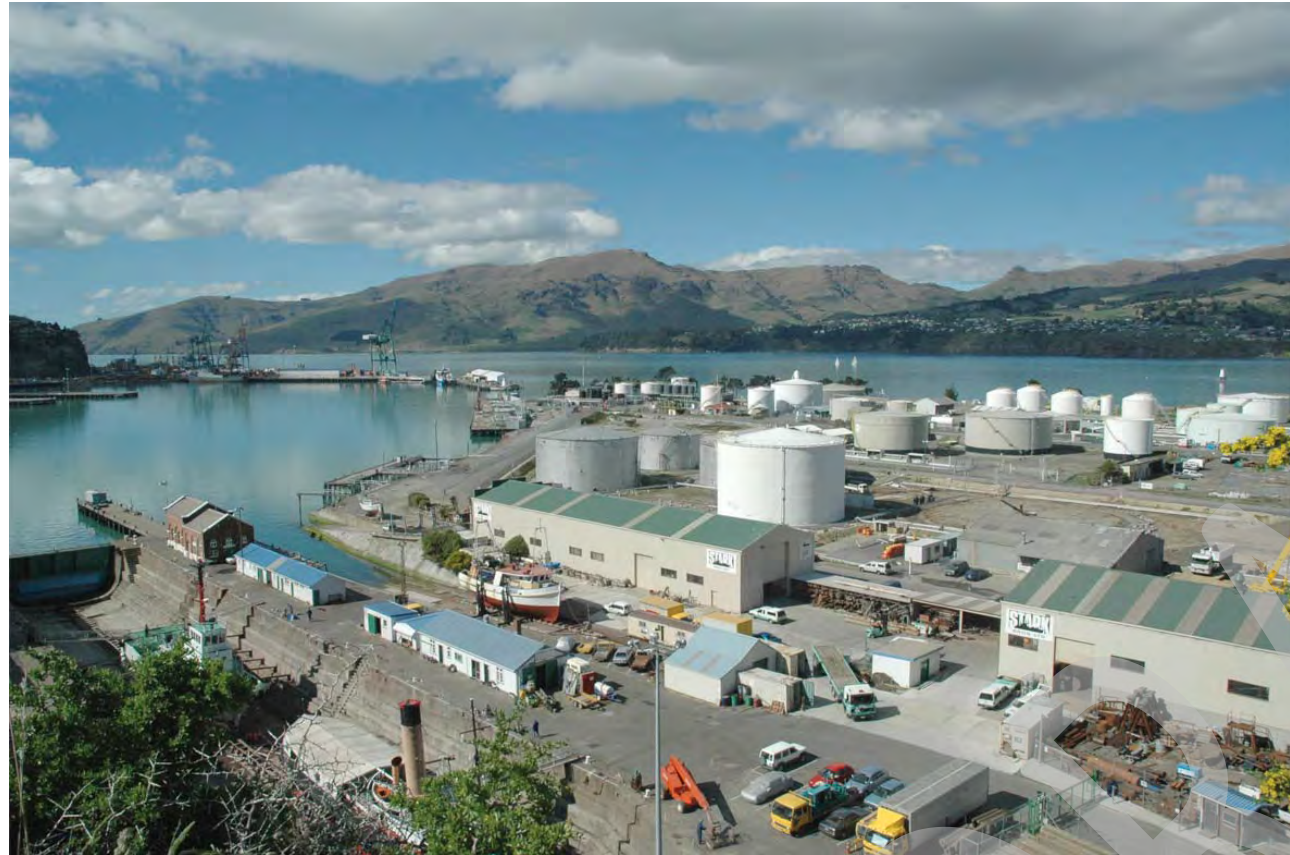
The coastline between Tapoa/Erskine Point and Battery Point has been heavily modified by Port industry
