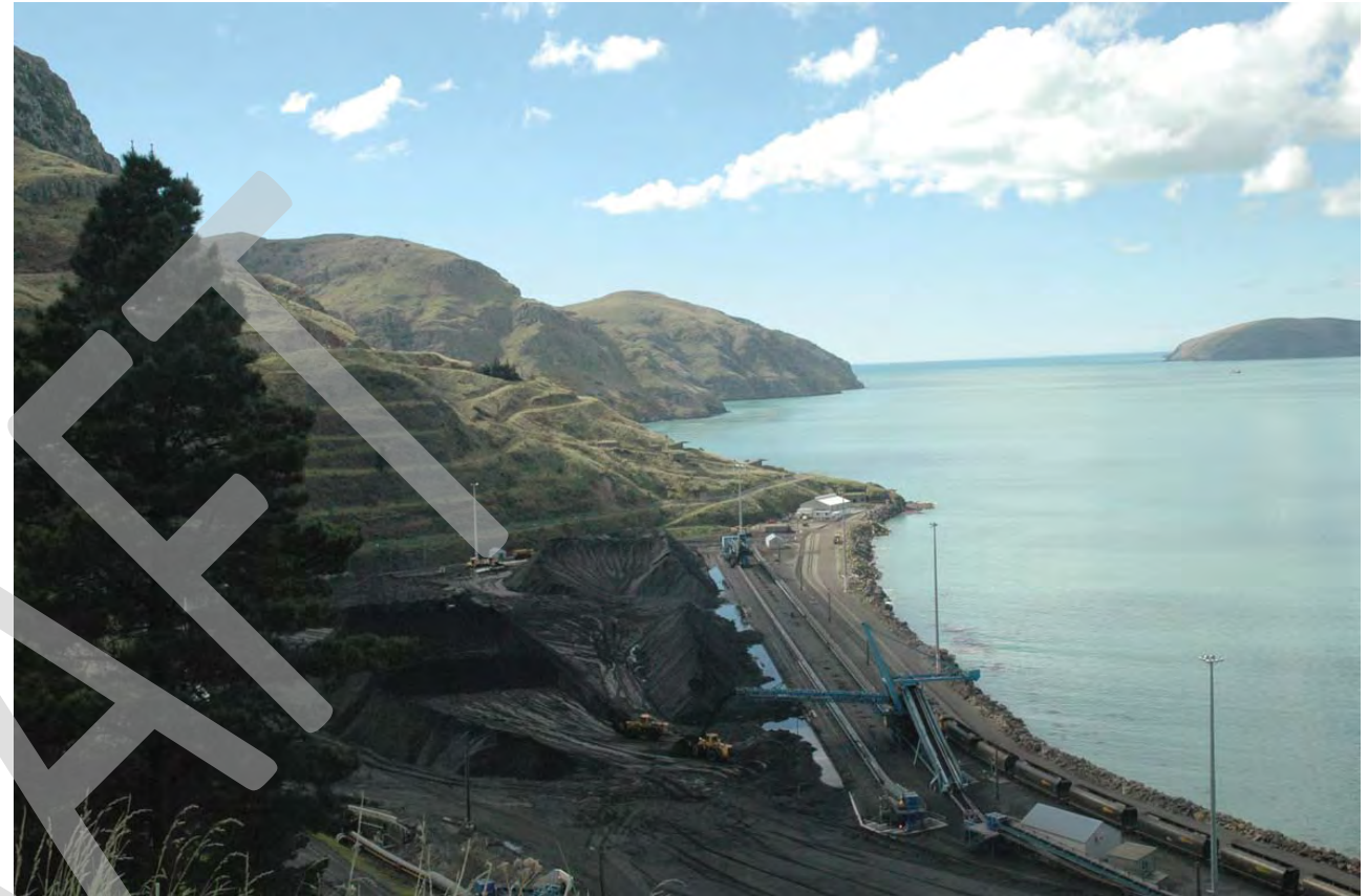
The reclamation required to create Cashin Quay, resulted the loss of little bays such as Buckleys Bay and Forwards Beach
