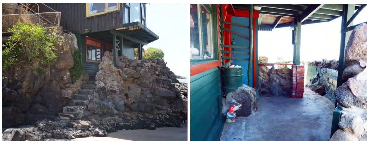
Photograph 4 & 5: Left, bach 56 steps, and right recreation path passing under the bach 56 upper story overhang.
