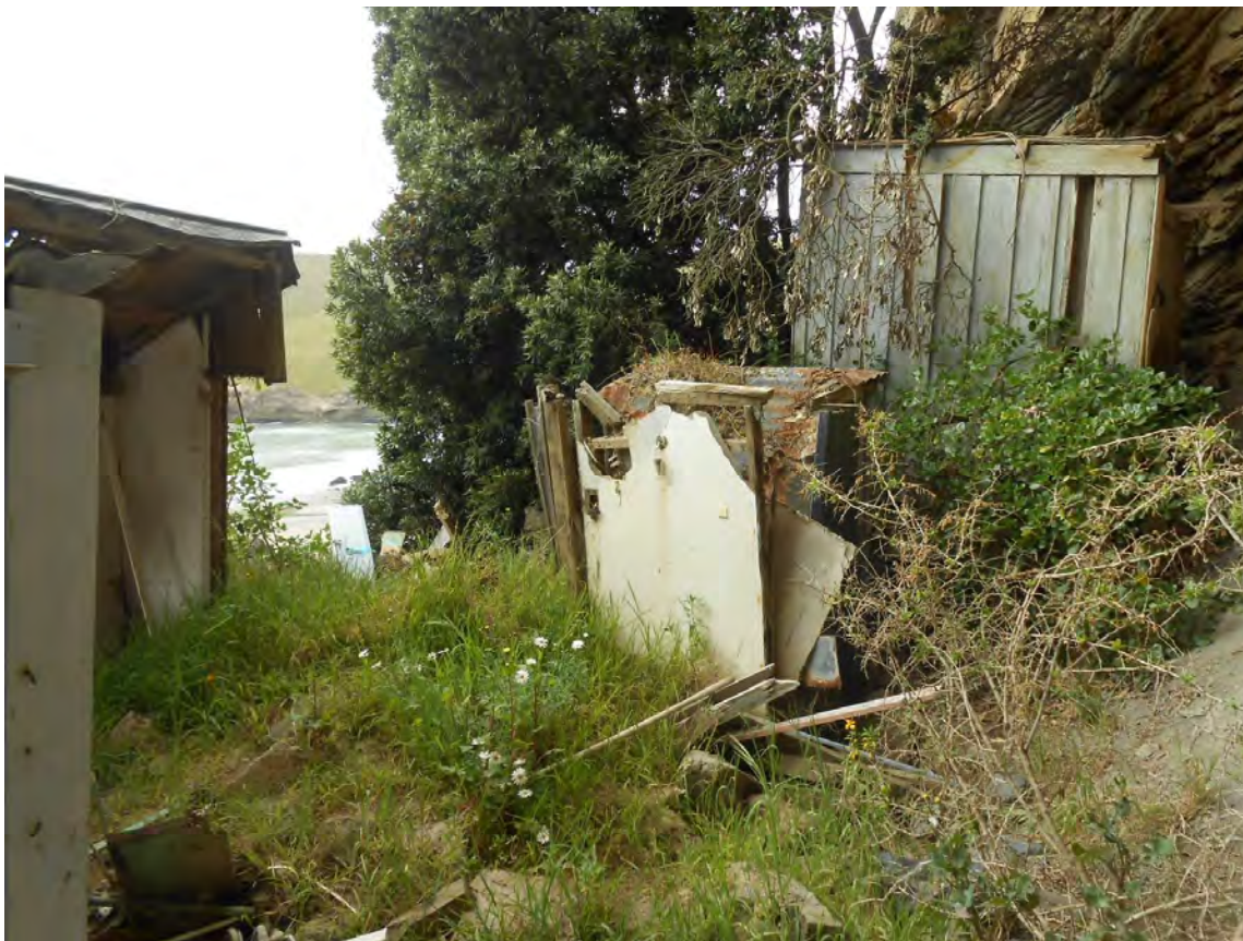
Destruction caused by rockfall debris hitting rear of bach at No.63 Hobsons Bay
