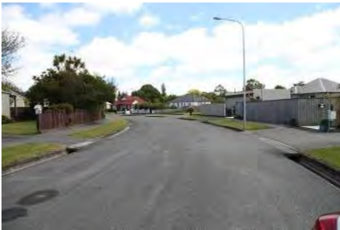
Piko Crescent Streetscape
