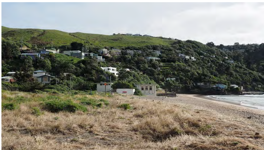
View of the existing LH zone from the foreshore
