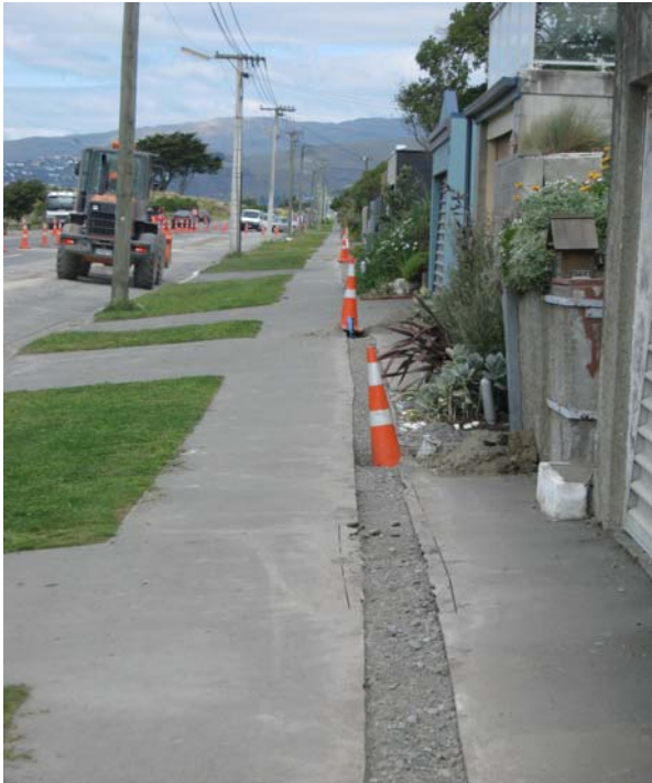
Marine Parade, Southshore, new water and sub-mains installation.
