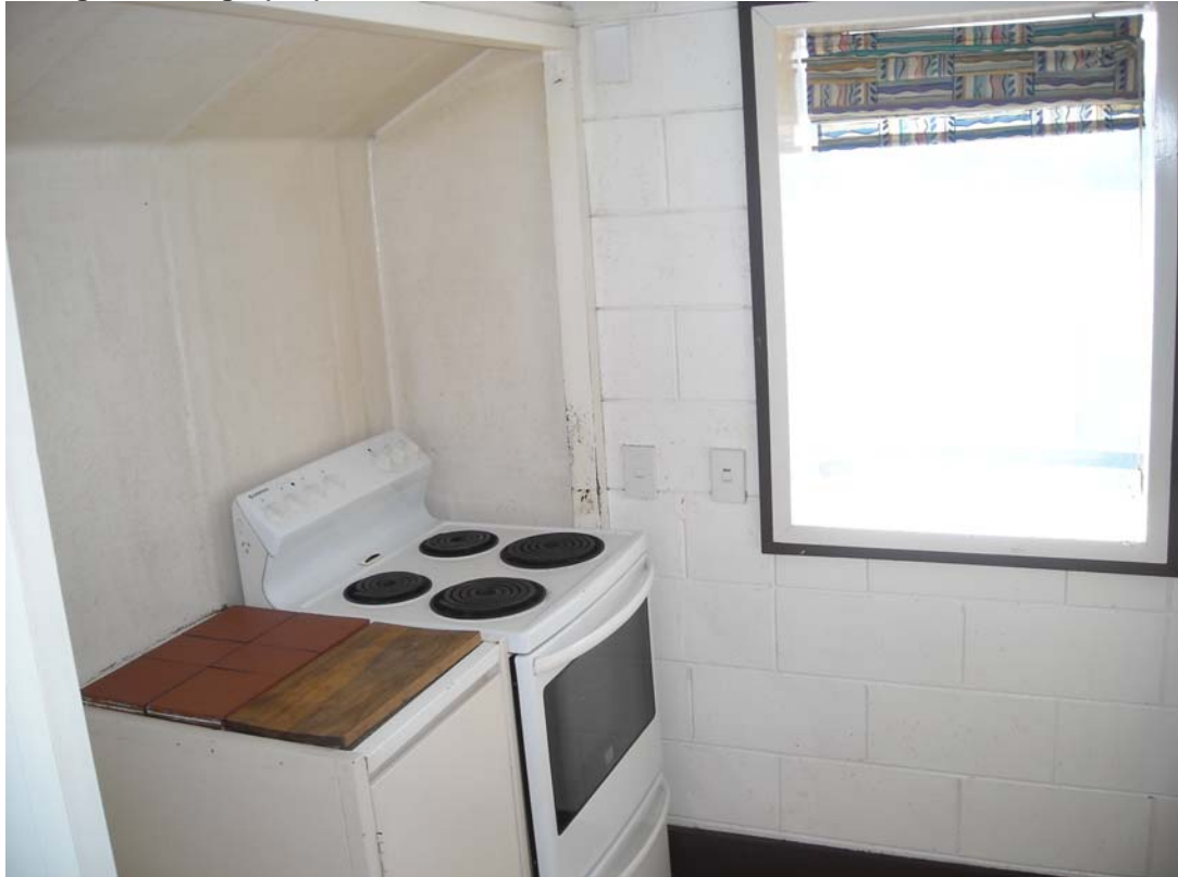
Unlined fibreglass wall in kitchen. Unlined concrete block walls.
