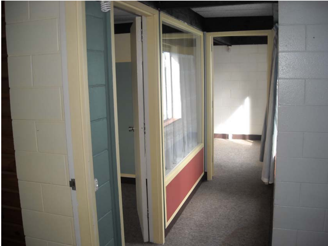
Typical interior showing unlined concrete block walls.
