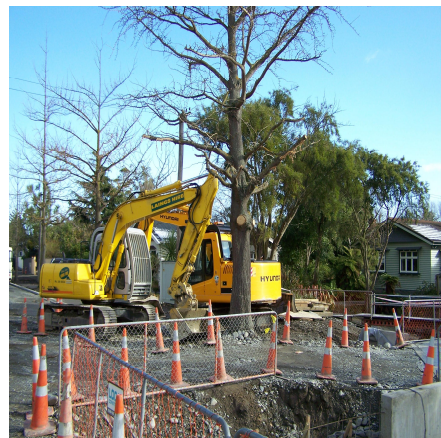
Photograph 8 Compaction and crushing of root plate by vehicles.
