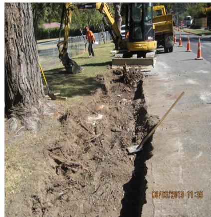
Photograph 6 Root severance by trenching with excavator.
