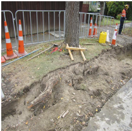
Photograph 5 Root severance by trenching with excavator.
