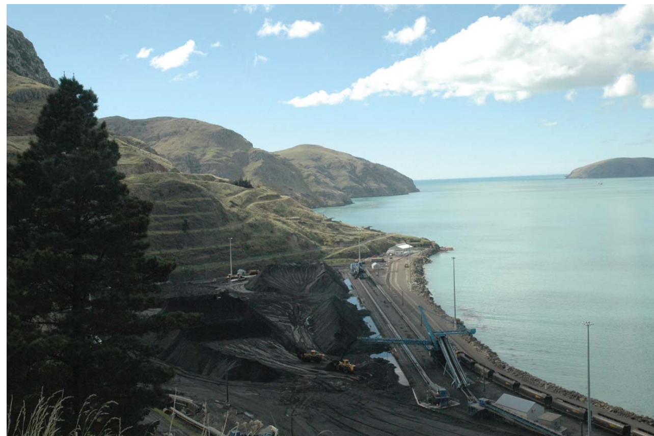
The reclamation required to create Cashin Quay, resulted the loss of little bays such as Buckleys Bay and Forwards Beach
