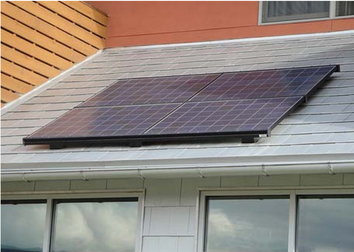
Flush mounted solar panels are generally visually less obtrusive as they blend in with the structures they are mounted on. Image Source: http://www.solardave.com/
