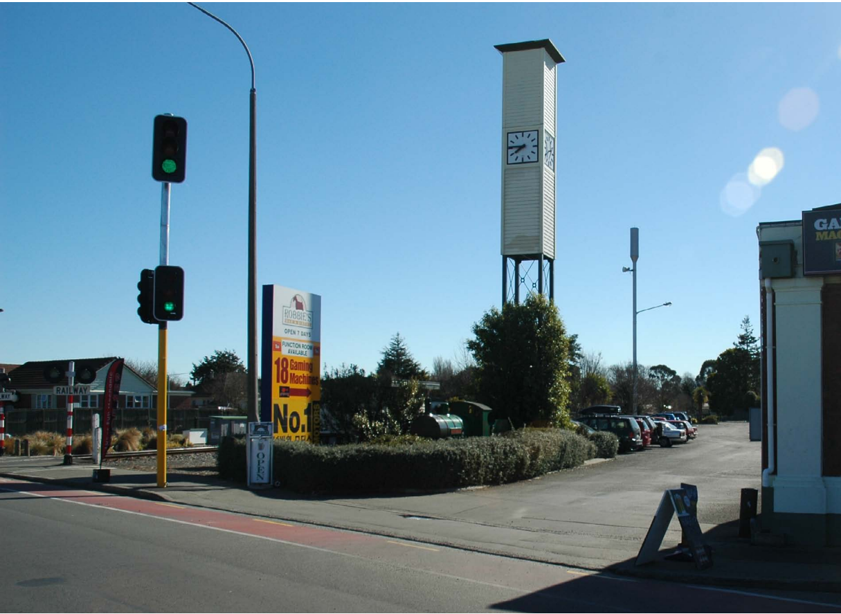
Telecommunication towers can be integrated into the landscape disguised as other structures such as this clock tower in Elmwood. This camouflage method is only appropriate in selected cases.
