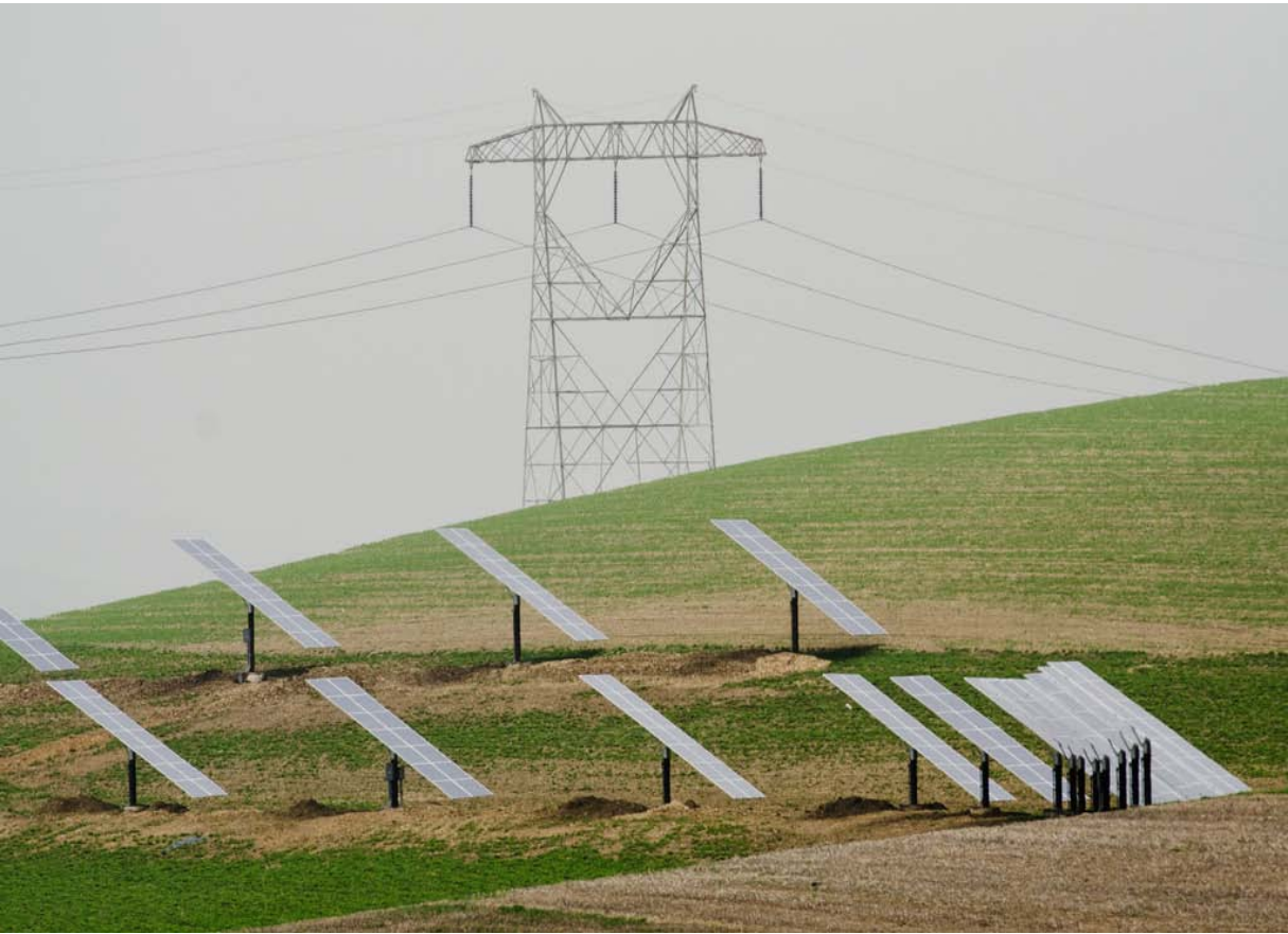
A small commercial solar farm with pole mounted solar panels . Image Source: Copyright U.S. Department of Agriculture 2011. This photo was taken on April 20, 2011 using a Nikon D7000. POLE
