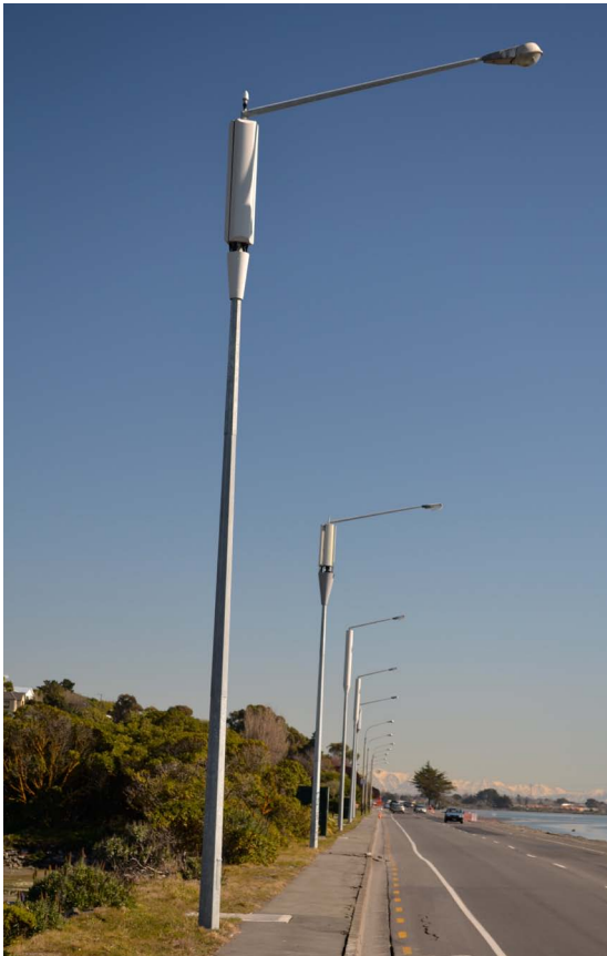
Clustering of cell phone towers and integration with existing structures is often preferable.
