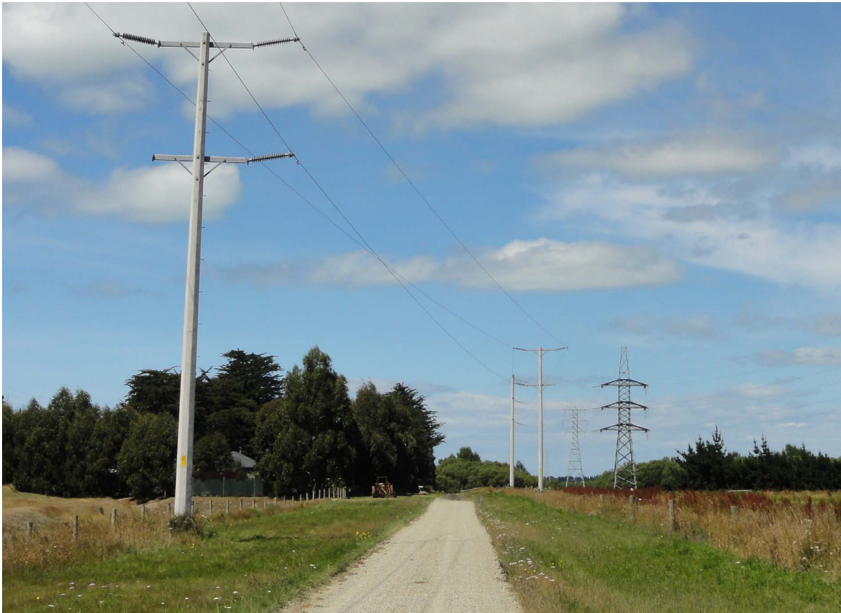
Due to their industrial appearance and bulk, lattice towers often have a higher magnitude of visual effects in comparison to single pole towers.
