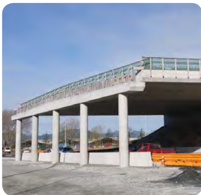
Construction of the Southern Motorway
