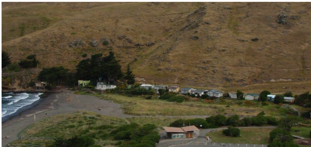
Overview, Taylor's Mistake baches. No.30 at left of photo; No.45 at right. No's 31-33 are in the trees at the end of the beach.
