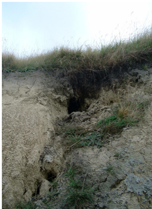
Tunnel gully exposed by earthworks
