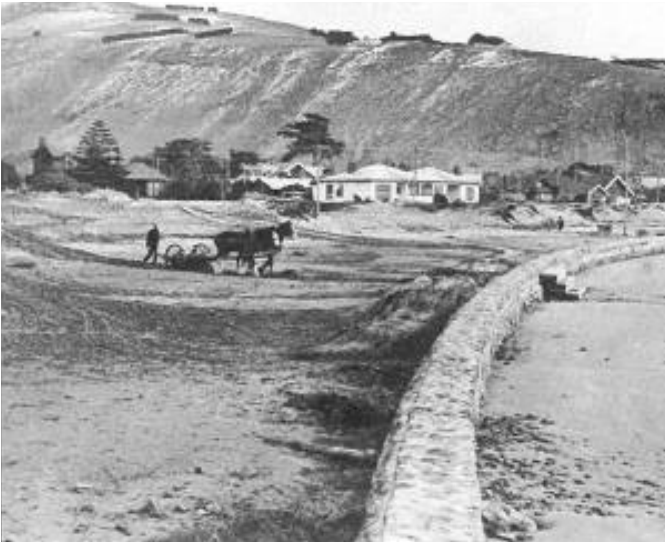
Figure 9. Sand hills being levelled and the new protective wall being reinforced at the Scarborough end of Sumner beach, 1931
