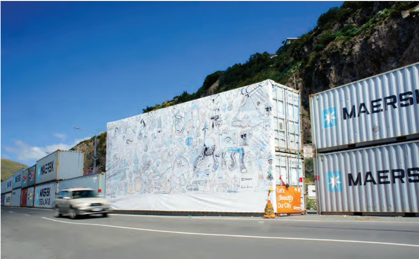
Figure 31. Containers placed for protection against rock fall along Wakefield Avenue
