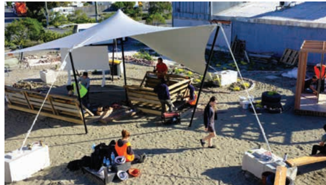
Figure 28: Photograph of the transitional project in Brighton Mall under construction
