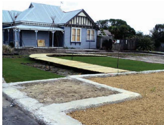
Figure 29: Photograph of the Greening the Rubble site on the corner of Beresford Street and Oram Avenue
