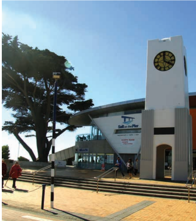
Figure 26: Photograph of the New Brighton Library
