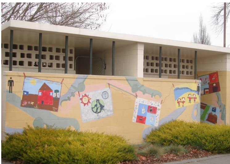
Figure 24. Toilet block on Worcester Street
