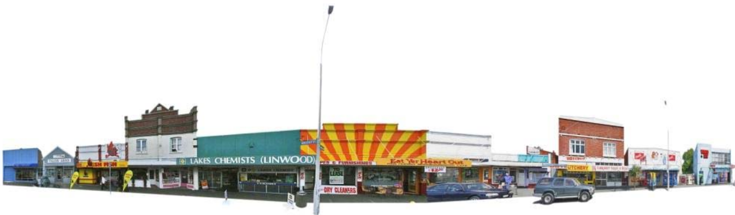
Figure 10. North-west corner of Worcester Street and Stanmore Road prior to demolition
