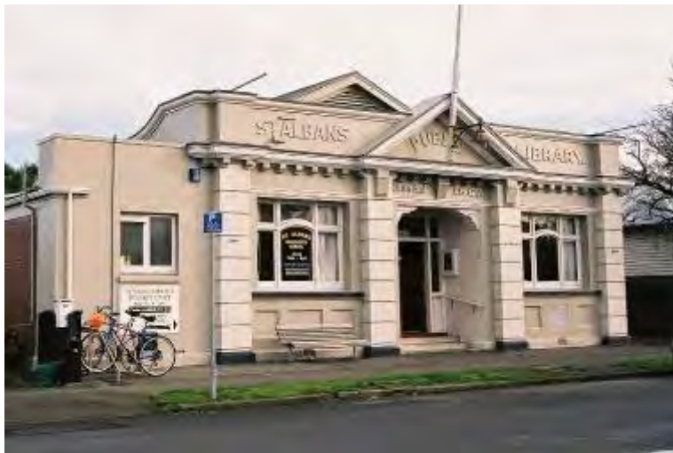
Figure 2c - St Albans Community Centre at 1049 Colombo Street (demolished 2011)
