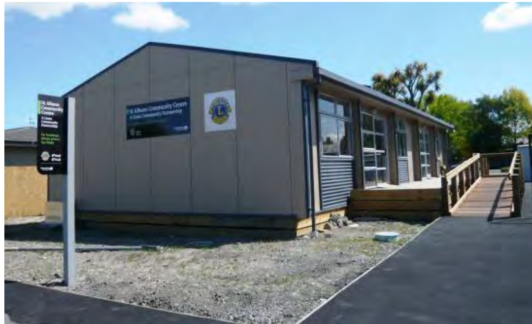
Figure 2l – The transitional community facility on Colombo Street
