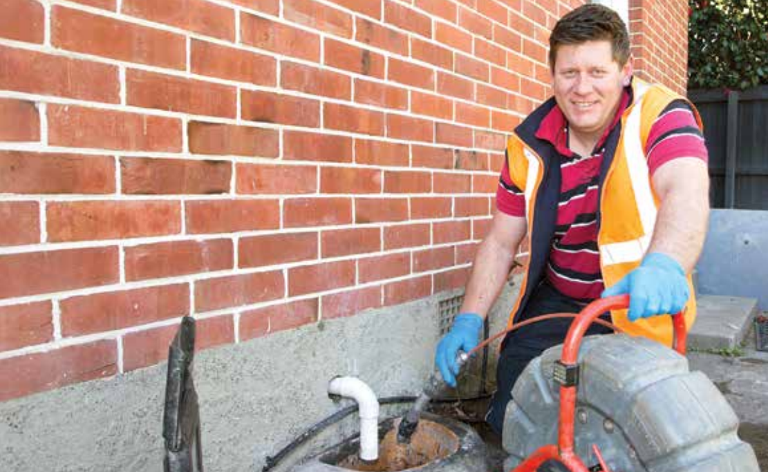
Homeowners are encouraged to use a registered drainlayer to check sewer pipes. Hamish Denny of Drainworkz uses a camera to check a home sewer pipe. Photo: Pam Johnson
