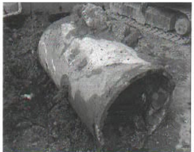
Photo 12 - Removed Section of Abandoned Stormwater Pipe
