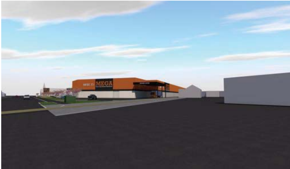
Existing Signage on Building (viewed from Harewood Road East)
