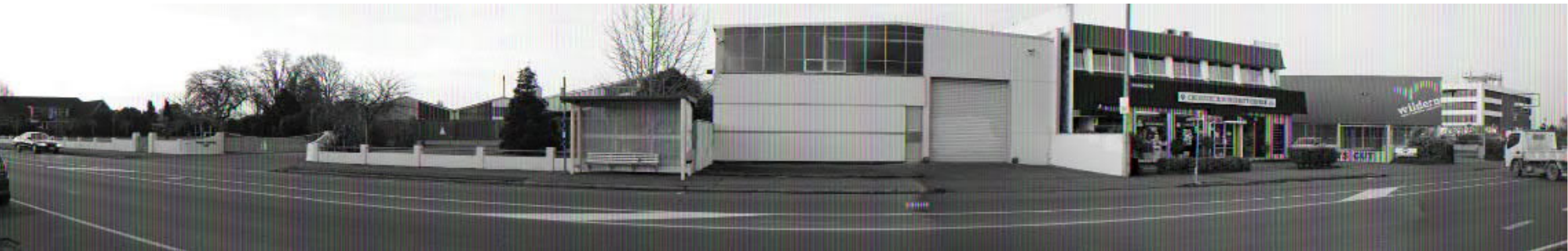
Image 4.3-Eastern End of Harewood Road Frontage: Showing existing urban character with varied building structures, carparks and security fencing
