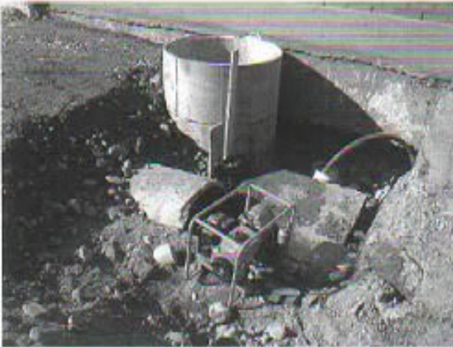
Photo 13 - New Sump to Block up Abandoned Pipes and Trap any Residual LFO from Migrating
