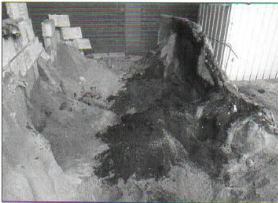
Photographs of the Removed Light Fuel Oil Tank and Containment Bunker at Sanitarium Health Food Company
