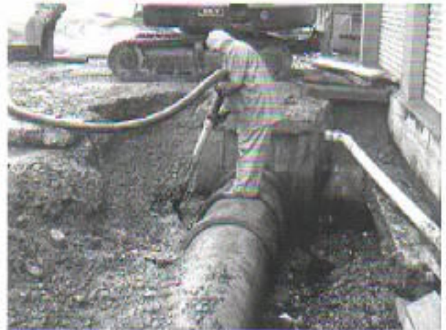
Photo 10 - Pumping out the Free Flowing LFO and Impacted Groundwater
