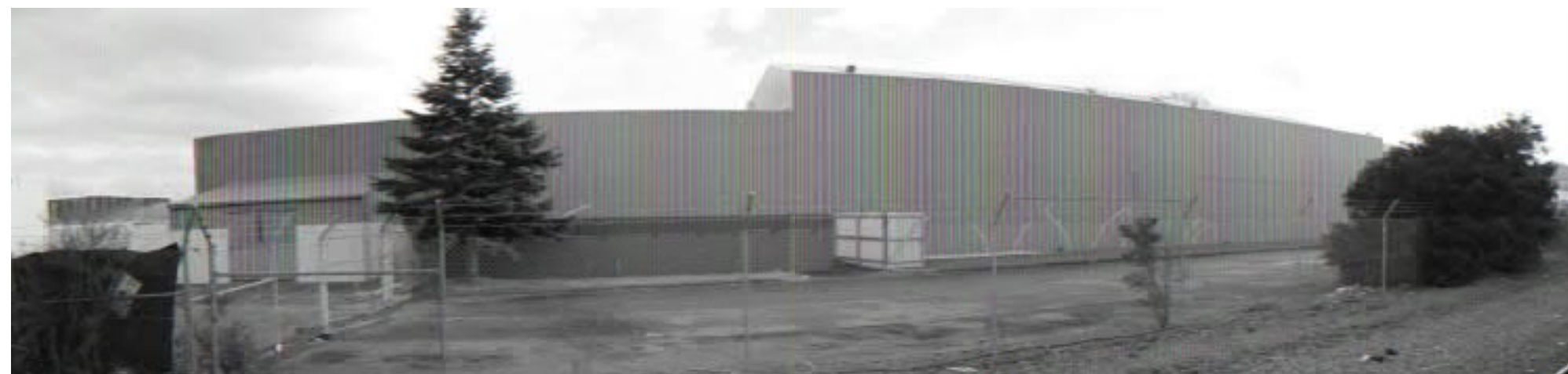
Image 6.7-Existing Hardstand Behind Factory:
