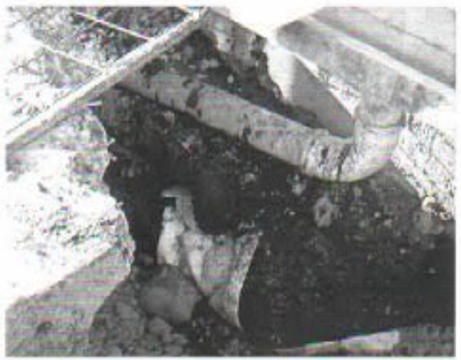
Photo 6 - Initial Contamination Identified by Sanitarium Staff
