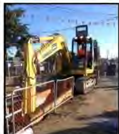
An example of open trenching
