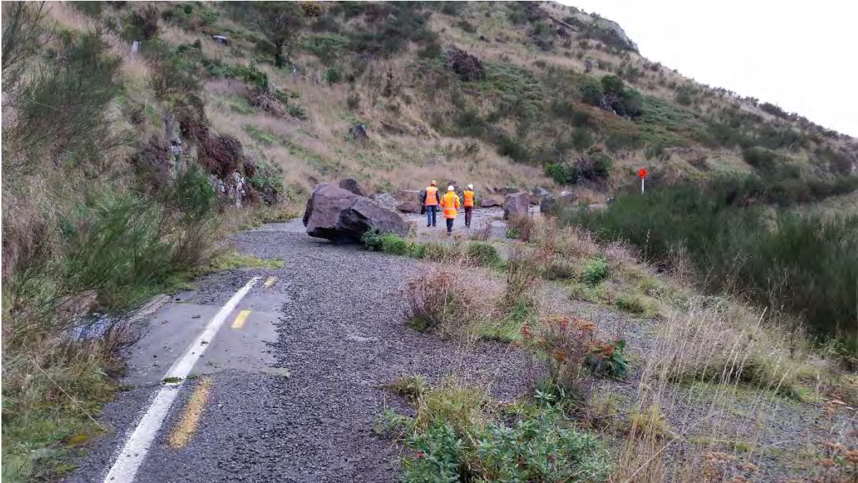
Figure 2.1 Closed section of Sumner Road, overlooking Lyttelton Harbour
