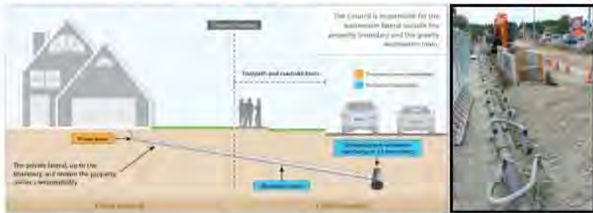
An example of a dewatering set up
