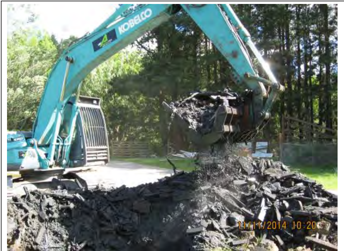
Demolition waste on Hororata dairy farm
