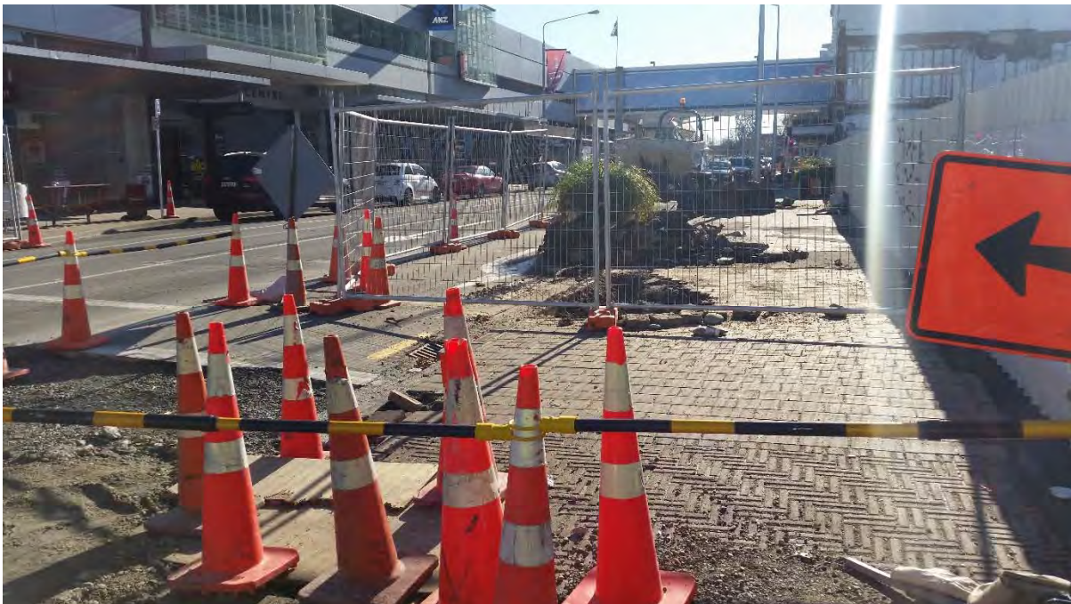
Figure 2.3 AAC First Phase Works, Lichfield Street
