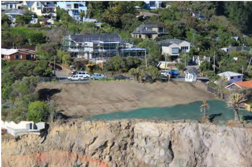
Slope stabilisation works on Port Hills site – hydro-seeding on cliff edge.
