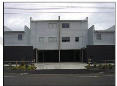
No ground level activity creates 'no mans land' along front boundary
