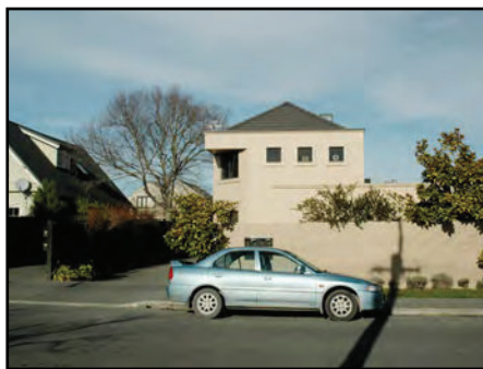
Poor natural surveillance from narrow street facades and small upper level windows
