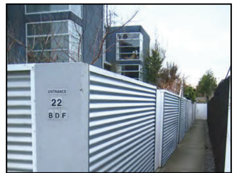
Narrow side boundary walkways are dark entrapment zones
