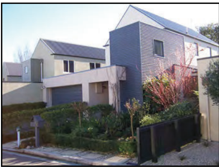
A semi-public landscape buffer zone is provided but no windows to monitor street level activity
