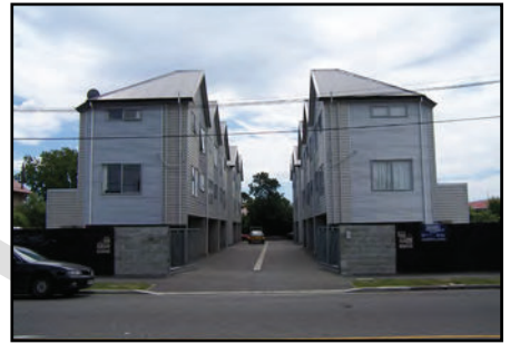
Direct facing windows across a narrow access way within a development
