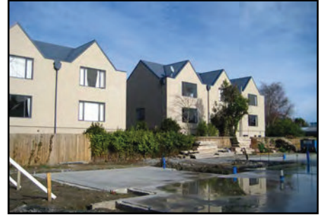
The extent of large windows facing side boundaries limits the options for future developments to avoid privacy issues
