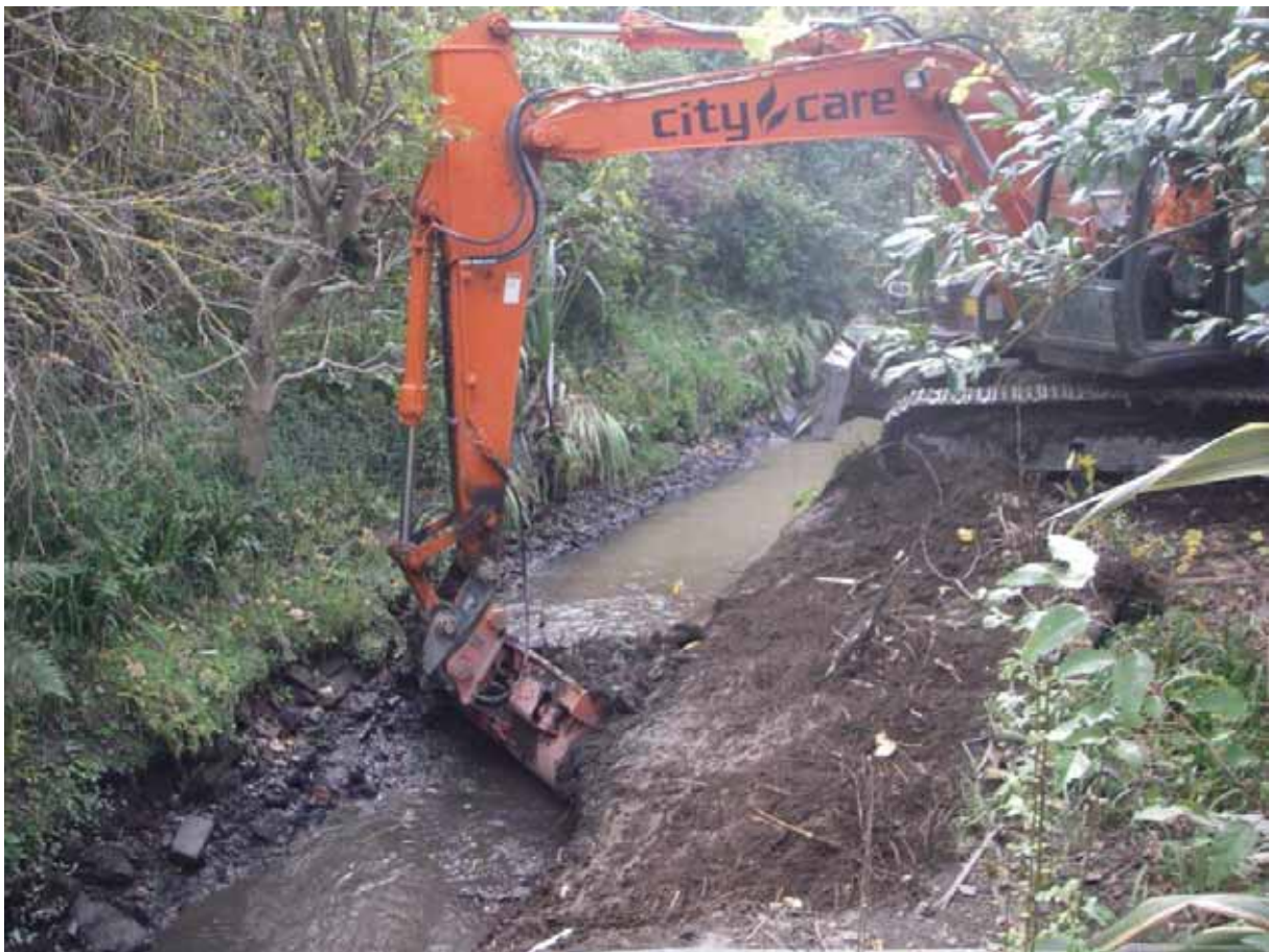
Figure 8 Maintenance works on Dudley Creek to increase channel capacity
