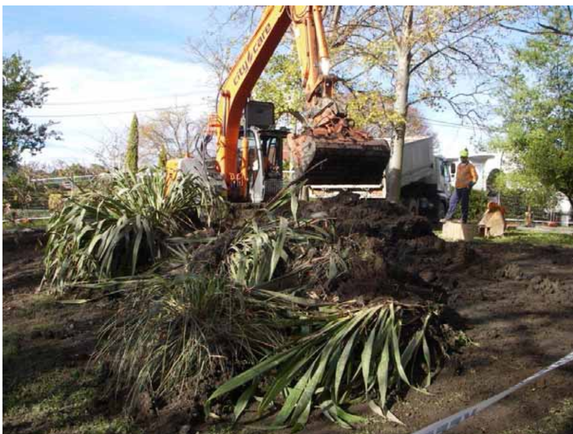
Figure 1 Clearing vegetation on Dudley Creek, May 2014
