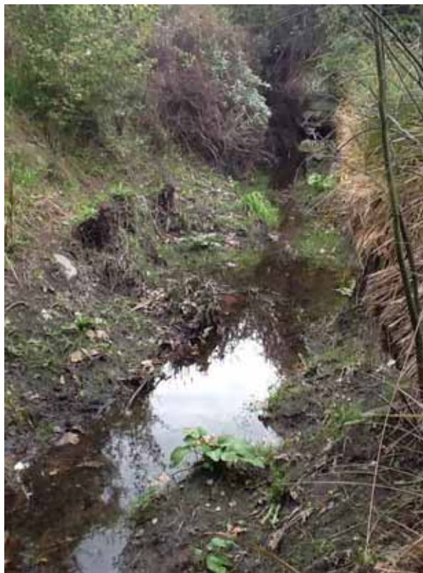
Figure 6 Upper Bells Creek – scope to increase channel capacity
