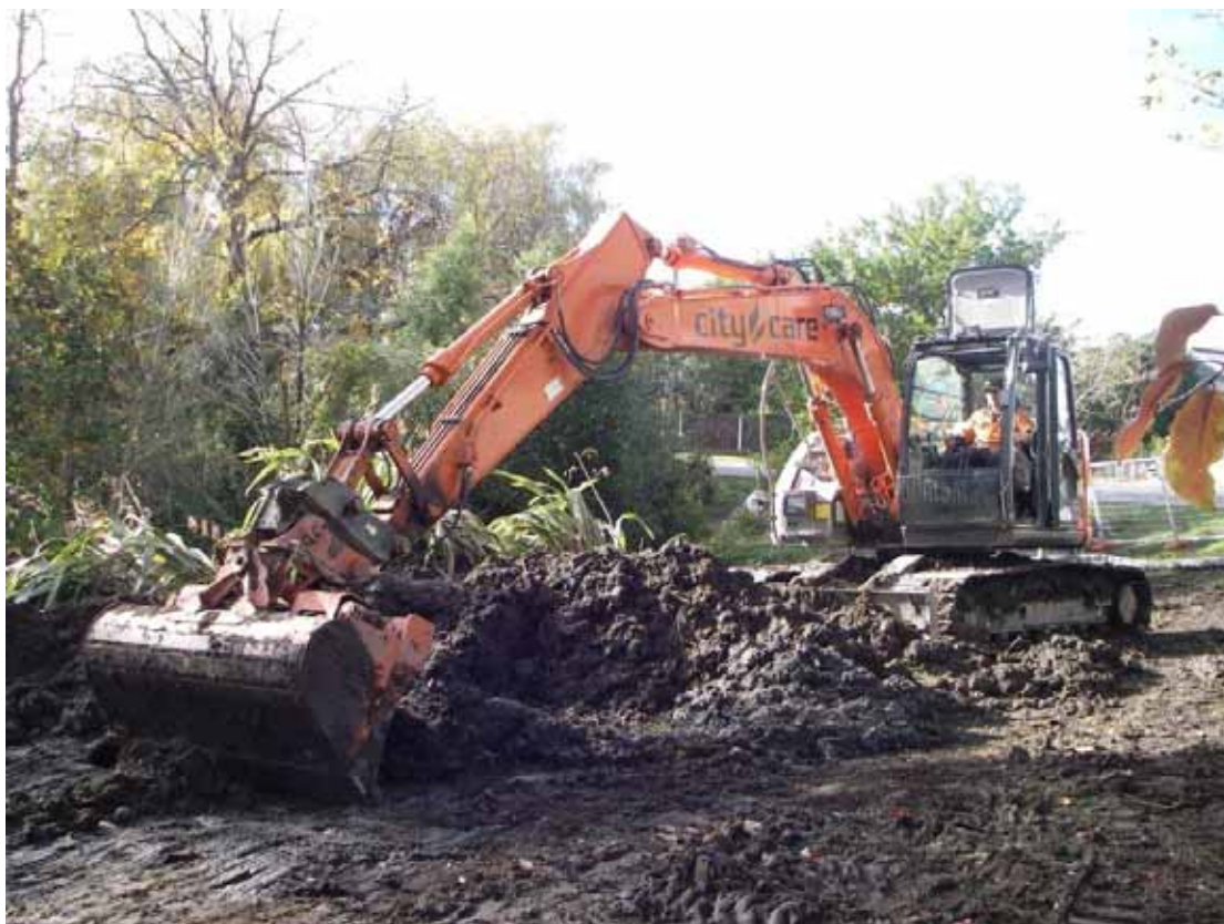
Figure 5 Maintenance works on Dudley Creek to increase channel capacity
