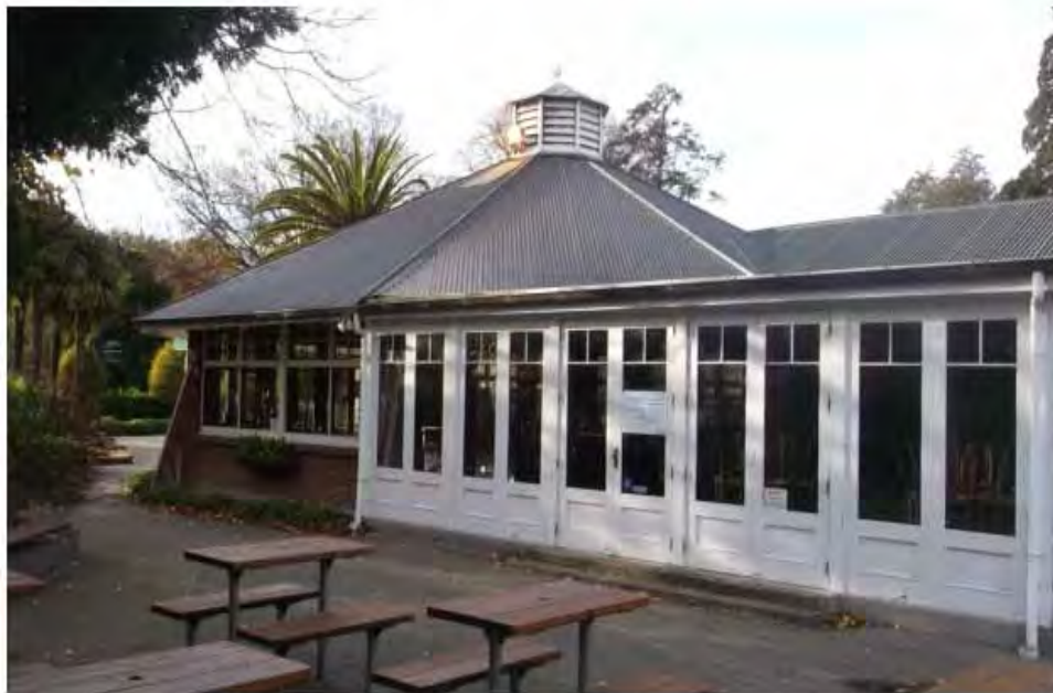
Photograph 2 – Tea Kiosk, Northern Side
