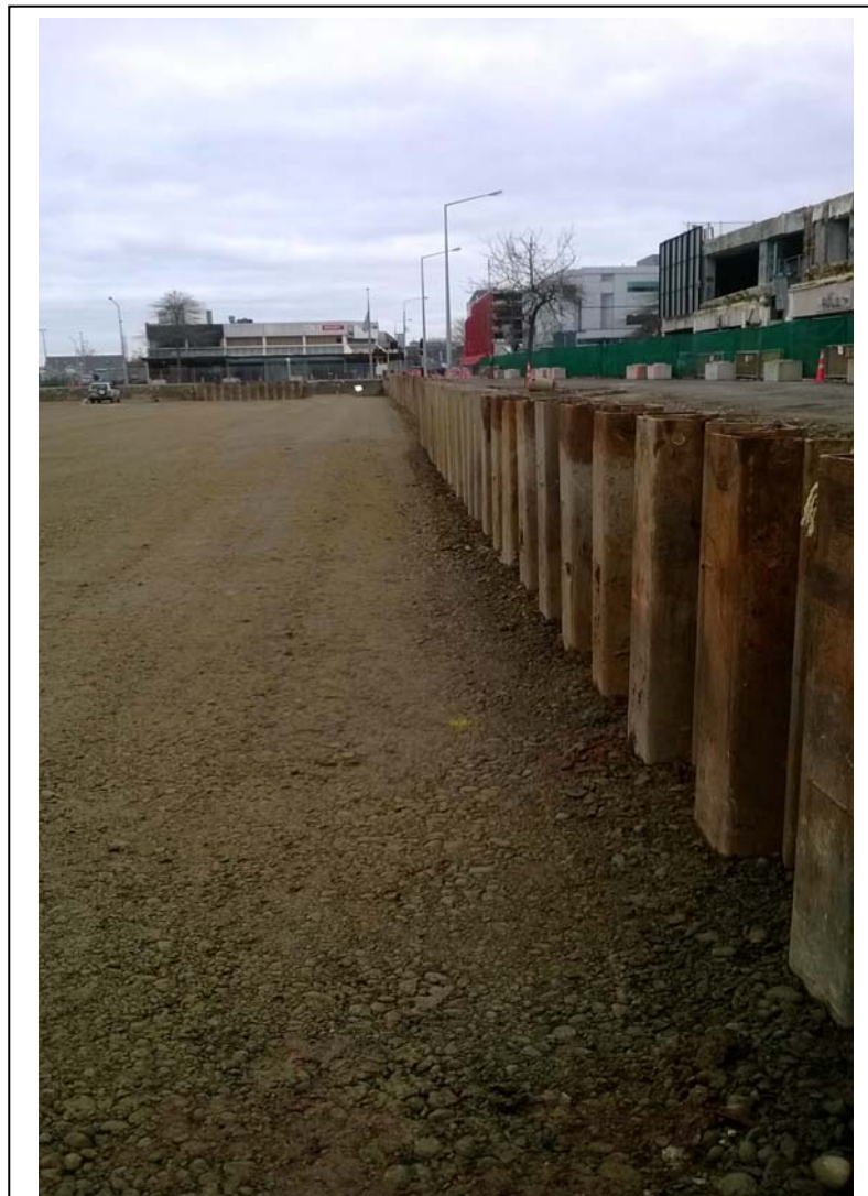
Transport Precinct final design levels.
