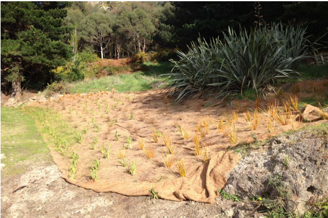
Use of Coconut Matting and Native Planting on CERA Port Hills Property
