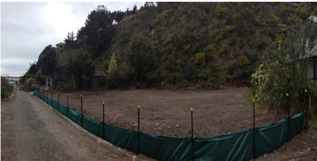
Silt Fence On CERA Port Hills Property
