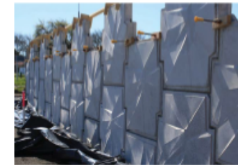
MSE RETAINING WALL DESIGN (PROPOSE TO MATCH WITH EXISTING CSM DESIGN - SUBJECT TO AGREEMENT WITH NZTA AND FULTON HOGAN)
