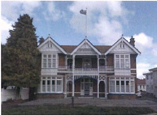
15. Number 52 Armagh Street. Pre-demolition (2009 picture).
