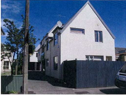
7. 49 Ely Street. An example of modern medium density development within the SAM.
