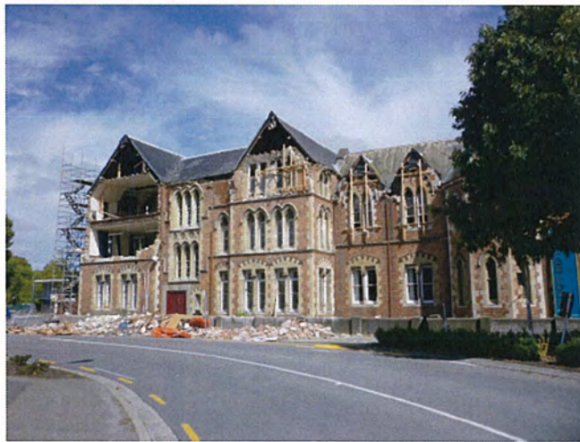
16. Cranmer Centre, number 32 Armagh Street. Earthquake damage and Pre-demolition (2011 picture).
