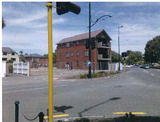
11. Number 338 Montreal Street (corner site). Adjacent to cleared site following demolition of no.52 Armagh Street (January 2013).
