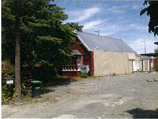
7. Number 25 Armagh Street. Adjacent to cleared site following demolition of Number 5 Cranmer Square (January 2013).
