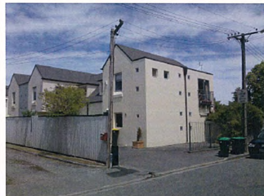
12. Ely Street. An example of modern development presenting a blank frontage to the street and with little vegetation.
