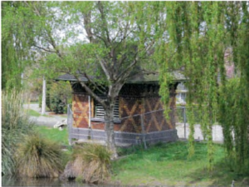
1. Oxford Terrace Pumping Station, City Plan Group 3 Listed Heritage Item.
