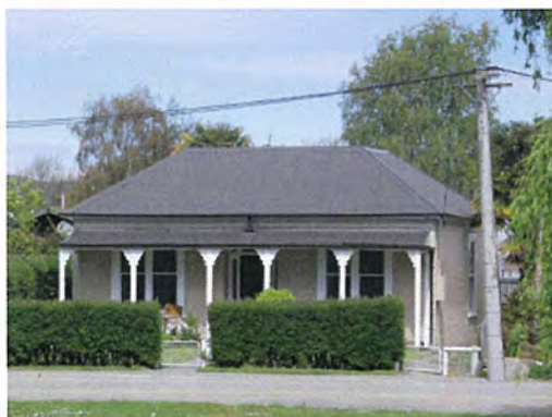
5. Number 396 Oxford Terrace photo showing example of a character property.
