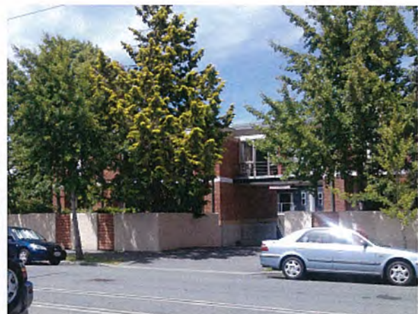
6. Armagh Street modern development.
