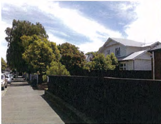
8. Gloucester Street. Wide building setbacks allow space for extensive mature vegetation.
