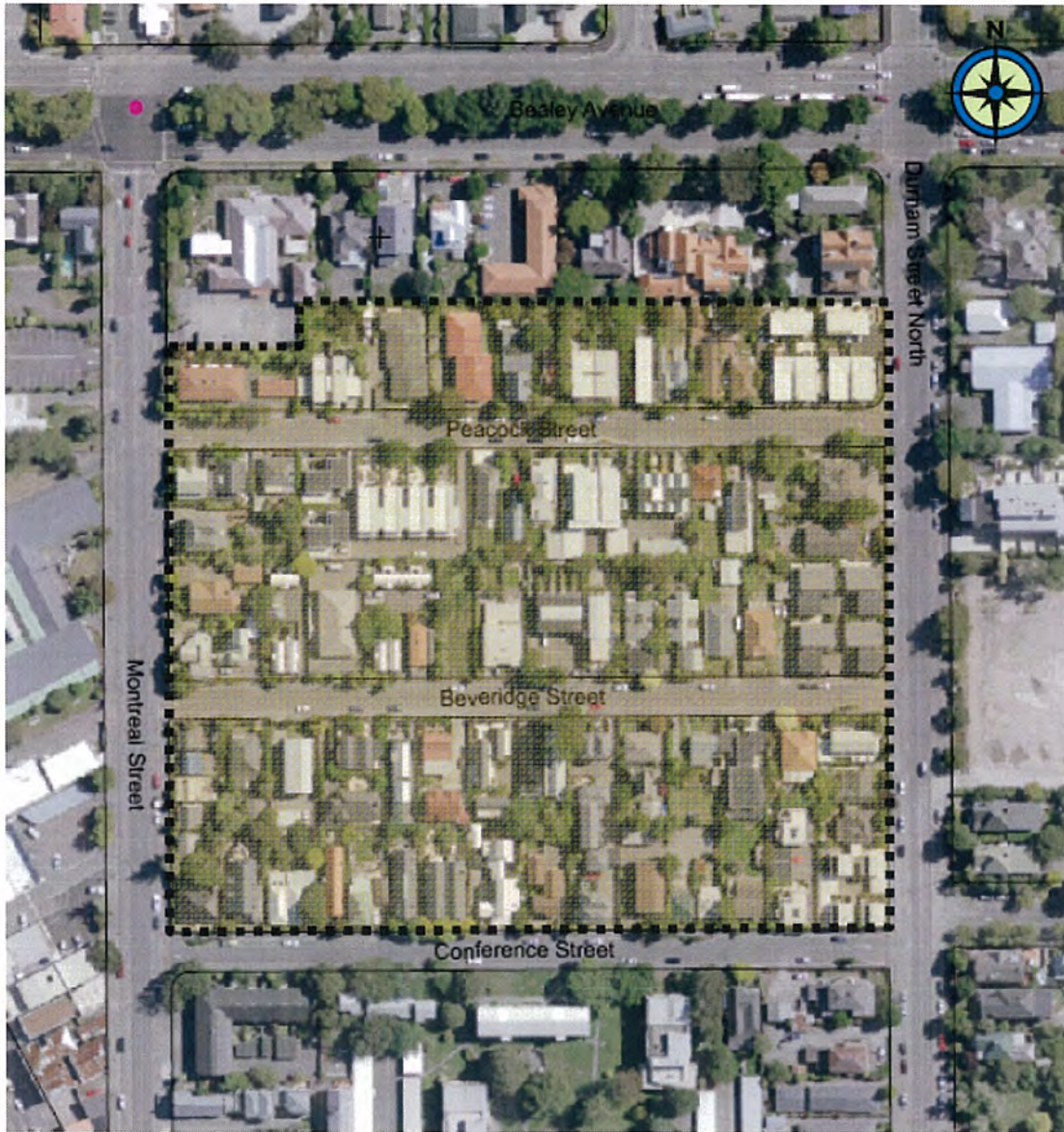
Attachment 3. Aerial photograph (2010) showing existing extend of SAM 26
