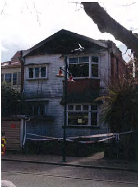
3. Number 33 Worcester Street, street scene. Pre-demolition, post-earthquake (also showing fire damage).
