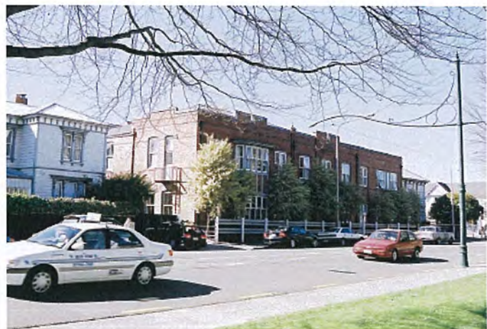
4. Flowers Building. Rolleston Avenue. 2004 photograph, pre-demolition and redevelopment.
