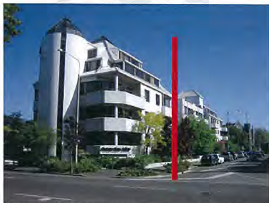
Chateau Blanc Apartments, west side of Montreal Street – area to the left of the line demolished
