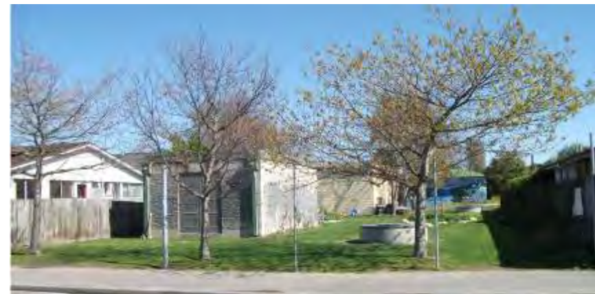
Figure 2j - Site used by Edgeware Village Green showing a number of site constraints – the substation, wellheads and pump station
