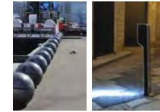
1. Distinctive, low-level lighting element. The main lighting treatment of the Coastal Pathway route. Intended to highlight the trail.
