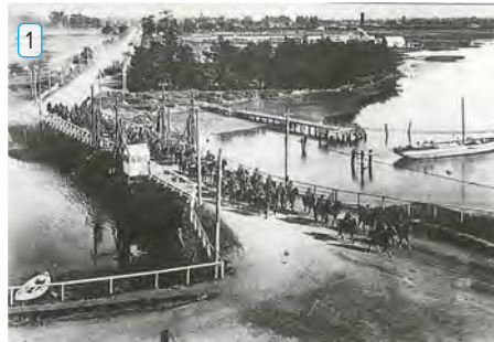
FERRYMEAD BRIDGE - DURING WW1 (SOURCE: 'THE ESTUARY, WHERE OUR RIVERS MEET THE SEA: DAVID BARR)
