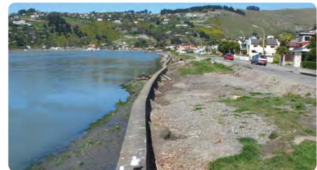
Figure 3.20 - The existing Beachville Rd seawall and space adjacent (Sept, 2012).
