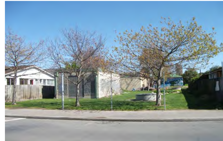
Figure 2m – Site used by Edgware Village Green showing a number of site constraints – the substation, wellheads and pump station.
