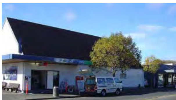
The building above does not address the corner or the street well with little visual interest, lack of active edge and visual interaction, in contrast to the neighbouring building.
