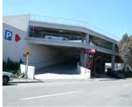
Compromised visibility of pedestrians for drivers exiting the parking building. Poor amenity for pedestrians resulting from the design of the ramp structure and building users.
