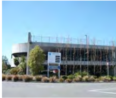
The introduction of a range of techniques, including design, landscape quality and site placement, can reduce the visual impact of car parking facilities.
