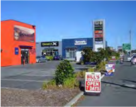
No demarcation of pedestrian access or space within the car park or adjacent to the building. Additionally, signage on the public footpath creating hazards for users.
