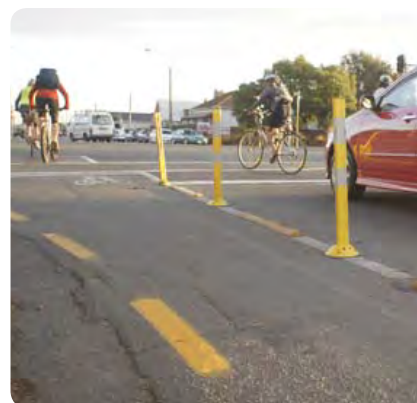
Top: Example of cycle lane markings and colour treatment through the intersection. Bottom: Example of vertical edge markers.
