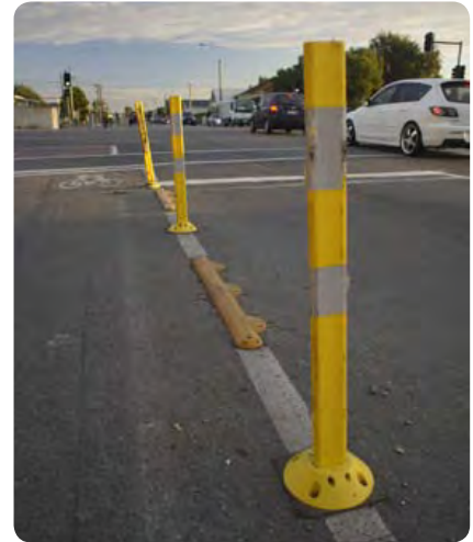
Example of a vertical edge marker.
