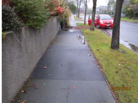
Photo 2 – Repair to footpath
