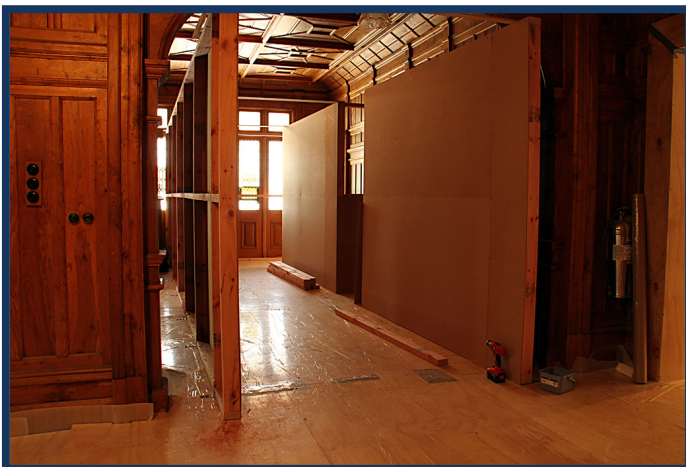
Pre Earthquake Repair Protection Works in Riccarton House Entry Hall.
