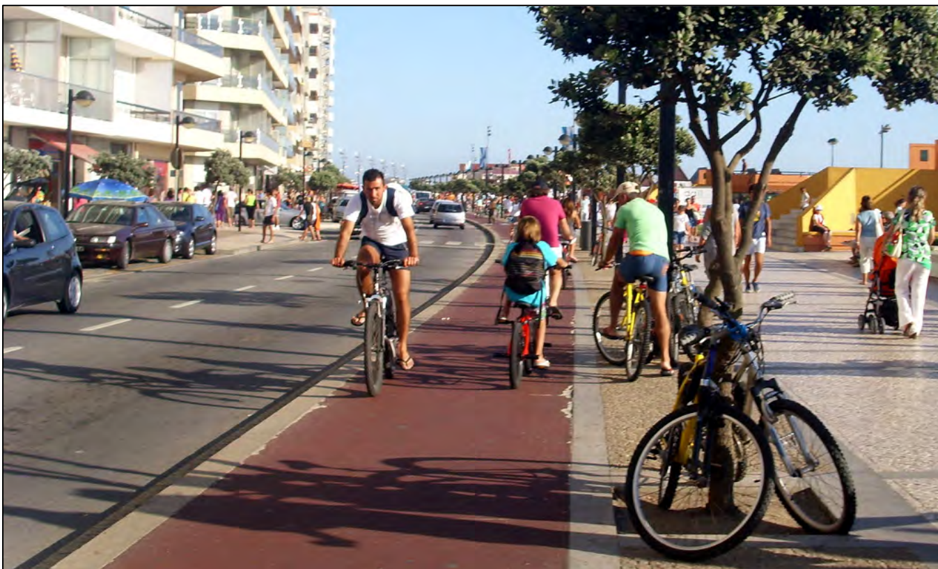
Figure 37: An example of how the kerb can be used to physically separate cyclists and motorists along the Póvoa de Varzim Waterfront in Portugal (Wikipedia Creative Commons license).
