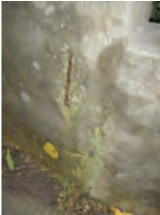
Damage caused by rusting reinforcing.
