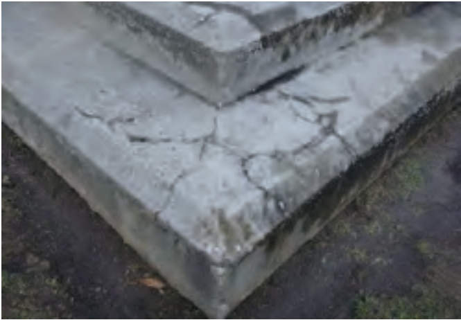
Base of monument showing cracking
