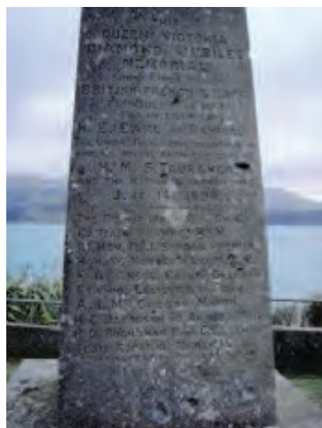
Pitting of stone. A substantive crack is also visible towards the right of the stone
