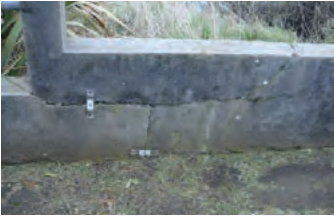
Cracks in concrete surrounding wall. Note “telltales”
